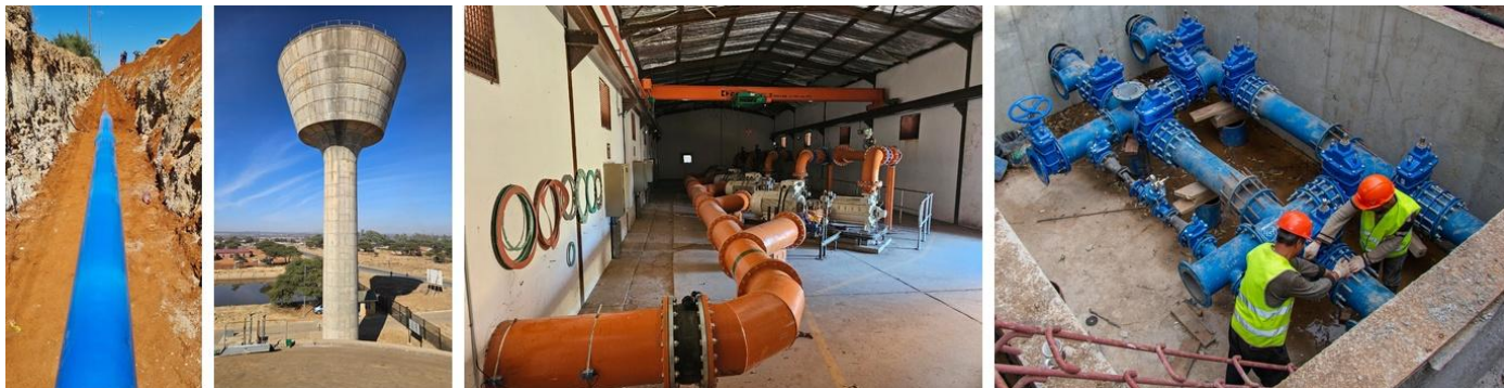
Bulk pipeline installation | Elevated storage | Pump station infrastructure | Valves and interconnections
